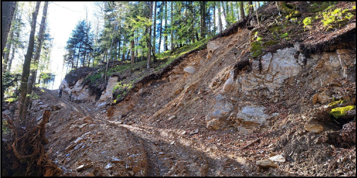
Top photo: ground visit of the logging site in April 2023, showing a large volume of wood being abandoned inside the forest. Bottom photo: deep logging roads are sometimes 4-6 m deep causing future erosion, April 2024.
